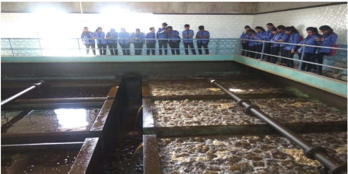
Rapid Sand Filter back washing procedure
